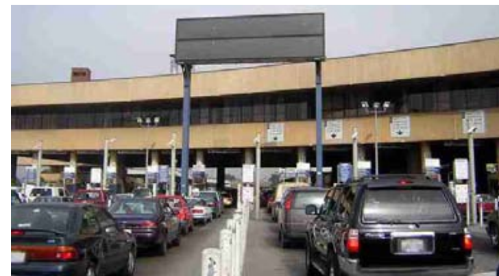
LPOEs vary widely in size, from very large ports to very small ports.
